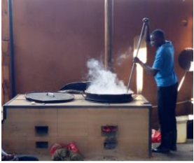
Institutional firewood energy saving stove at Victorious Primary School, Kampala Photo: Kimbowa R.
